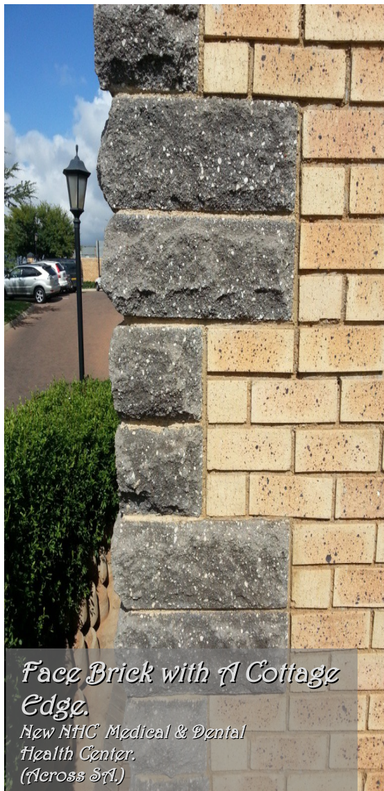
Fair Face 200 Series. This Project required a 20 Mpa Rating. A More Cost Affective to rainforest Walls. (Stefanutz N 12 Bridge)
